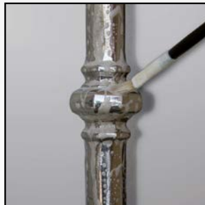
Application of the De-rusting product E4051/D: all polluted parts must be covered
